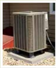
the winter they provide very comfortable and efficient heat until the temperature drops below the set point (usually 20 degrees F). Then the modulating plenum heater kicks in and works with the heat pump for extra savings. When controlled, a gas furnace kicks in.
